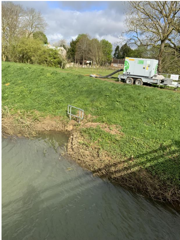
Photo 11 EA Trailer pump and flap valve asset adjacent to the bridge and sandbags deployed dyke side of flap valve
