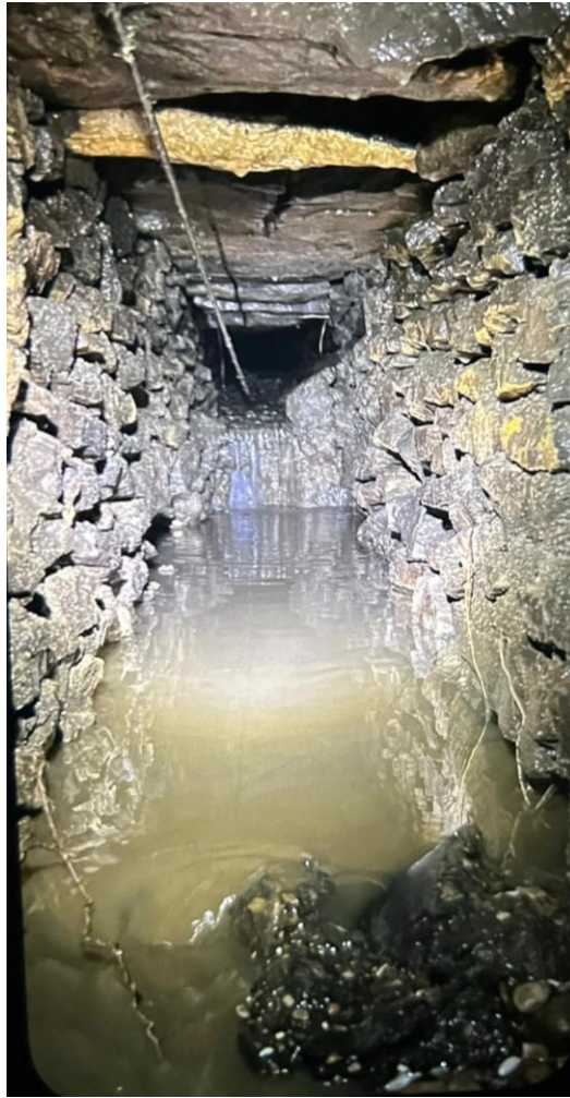
Photo 10 Tallington Surface Water Drain after cleansing
