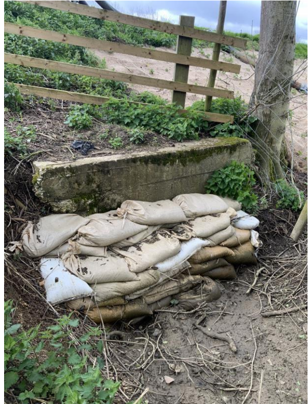
Photo 9 EA Trailer pump and flap valve asset adjacent to the bridge and sandbags deployed dyke side of flap valve
