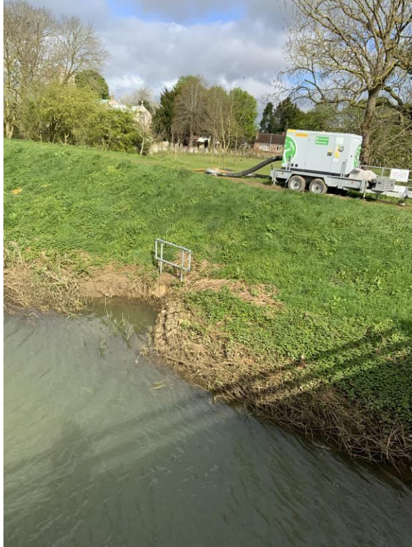
Photo 9 EA Trailer pump and flap valve asset adjacent to the bridge and sandbags deployed dyke side of flap valve
